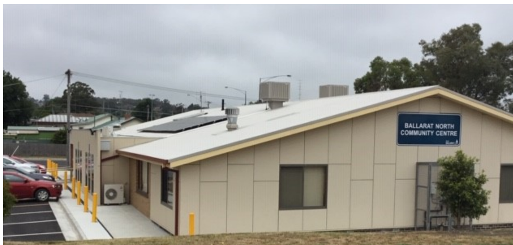
New evaporative coolers after being installed at Ballart North Community Centre
