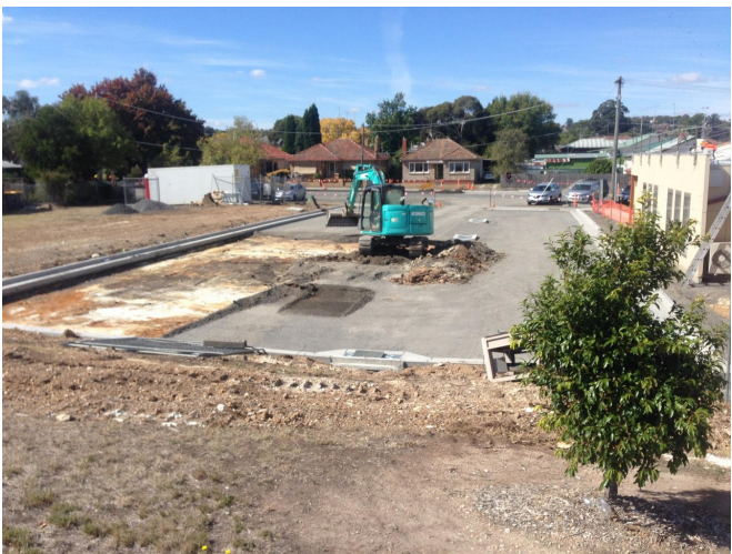
Delay at BNCC carpark due to water seeping up thru the base materials had to be dug out and replaced
