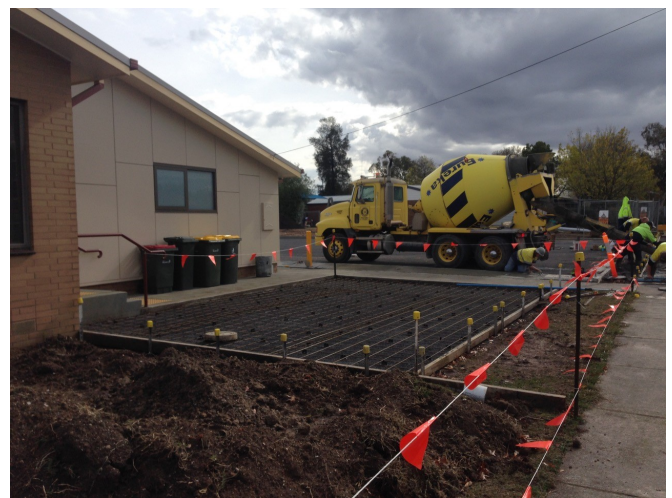
The last of the concrete goes in to the new bike rack area at BNCC
