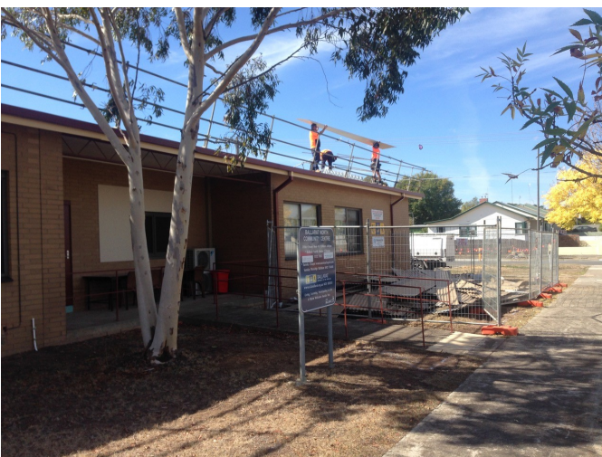
New roof on in 4 days at BNCC over the Easter break
