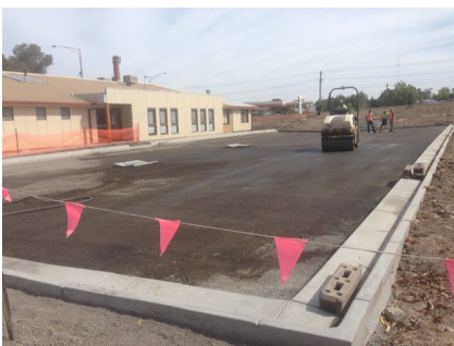
CoB putting the final touches on the blue metal base in the carpark today 5 April - next the bitumen to finish the job
