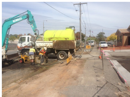
Just add water - and the BNCC carpark is ready for the final layer of bitumen 5 April
