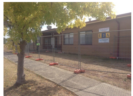
One project ends and the next begins on Monday 8 April - the removal and re-roofing on BNCC
