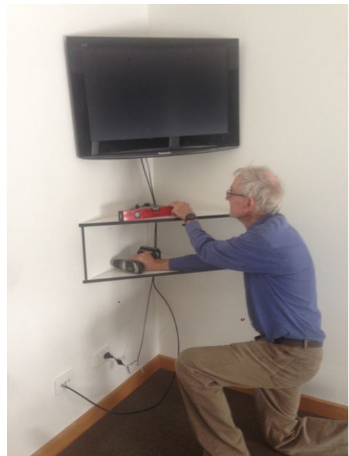
Terry Dixon doing his "woodworking magic" installing the new shelves in the BNCC Yellow and Green Rooms Friday 5 April
