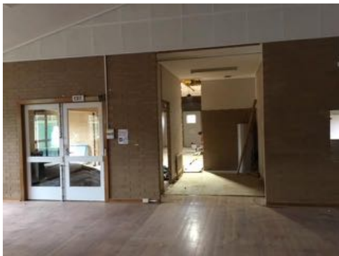
Construction at BNCC
